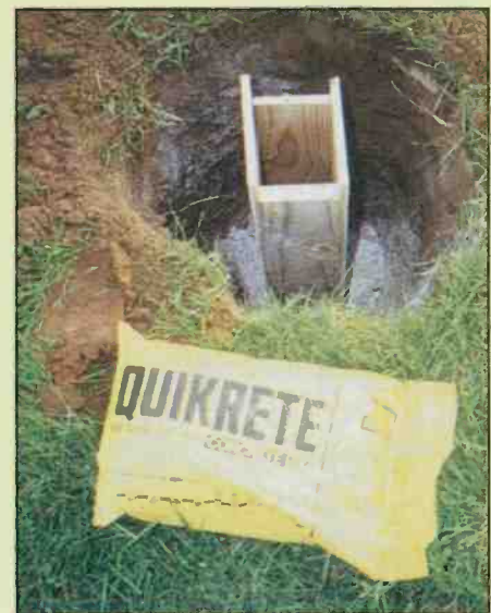
If you decide to mount a panel in the ground, be sure the buried cement wall is large enough to withstand the stress of your pole-mounted panel.
