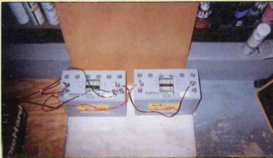
These two Deka batteries are sealed gel cell models and are maintenance-free. Notice the heavy-duty wiring that connects the batteries in parallel.
