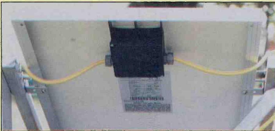
A panel's junction box showing a short outdoor extension cable going to another panel, and the other cable to the charge controller.
