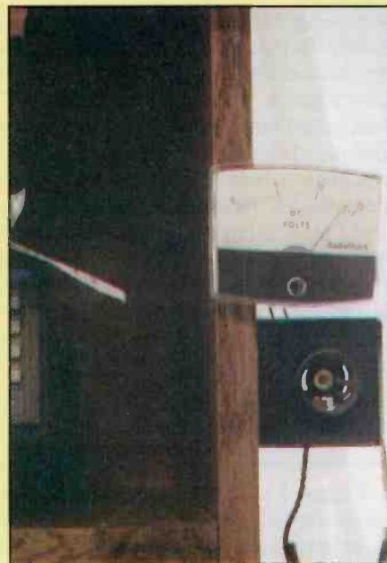
Inside the shack, the meter measures DC voltage and below is one receptacle providing free 12 Vdc power!
