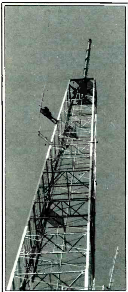
Installing an Army MARS receiving antenna 375 feet up, WDLI-TV transmitter tower located in Canton, Ohio. (Photo by John S. Papay, K8YSE/AAR5WI)
