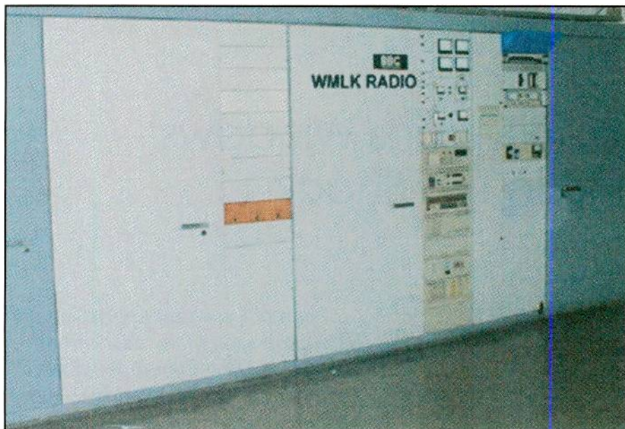
A 250-kW transmitter, now installed at WMLK, was previously in use by the BBC. (Thanks Charles Maxant, WV)
