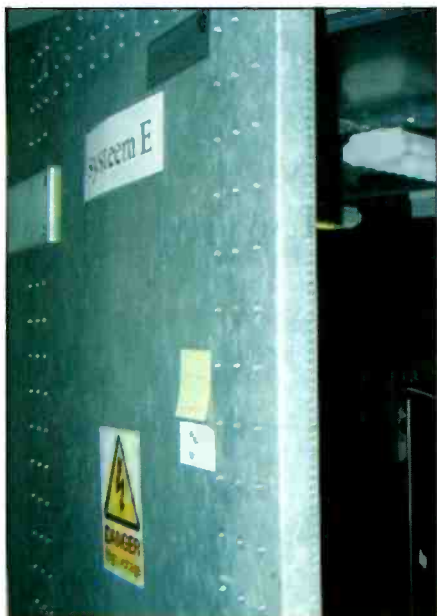
Here's a Faraday shield that encloses an entire room. Note the connection points along the edge of the door that ensure a complete electrical connection of all surfaces. No matter the size of the "box," the same principles apply. What you build will be just as effective as the professional model, as long as you take your time and follow the instructions provided in the column.
