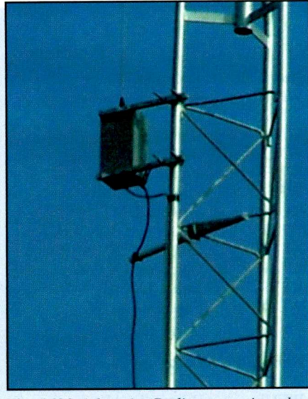
The 1690 Adventist Radio transmitter box is shown here with whip antenna mounted on a tower.
