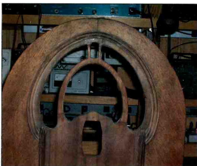
Photo K. Here's the finish layer of veneer in place and stained to match. It's starting to look as good as new at this point, thanks to some final sanding and trimming.
