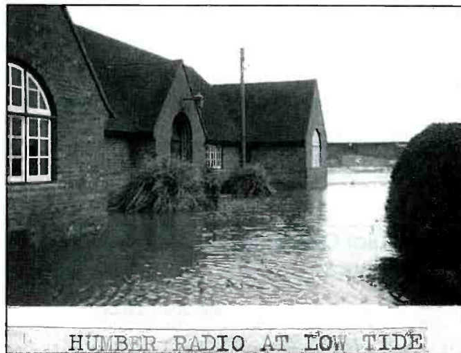
This is a shot of Coastal Radio station GKZ after the great storm of 1953 at low tide! As shown in last month's column, the interior was completely flooded.
