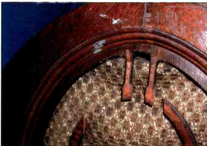
Photo F. It looks bad, but it is really worse than it looks. What remains is the center core of the fretwork, the outer layers are missing on both sides. A lot of work is needed.
