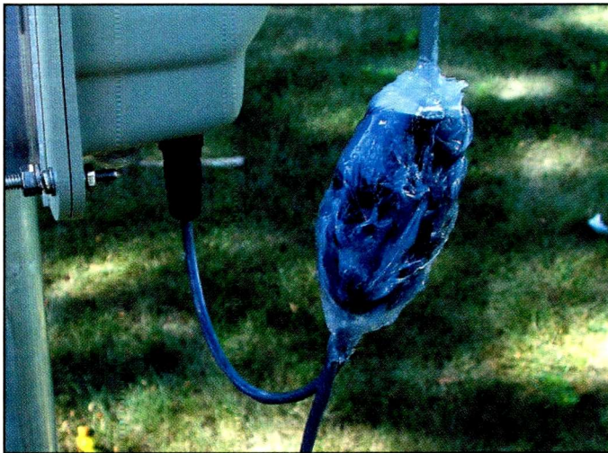
The plug portion of the wiring harness is taped, then covered with silicone sealant (not included) to protect it from the harsh outdoor elements. It's then taped securely to the boom.
