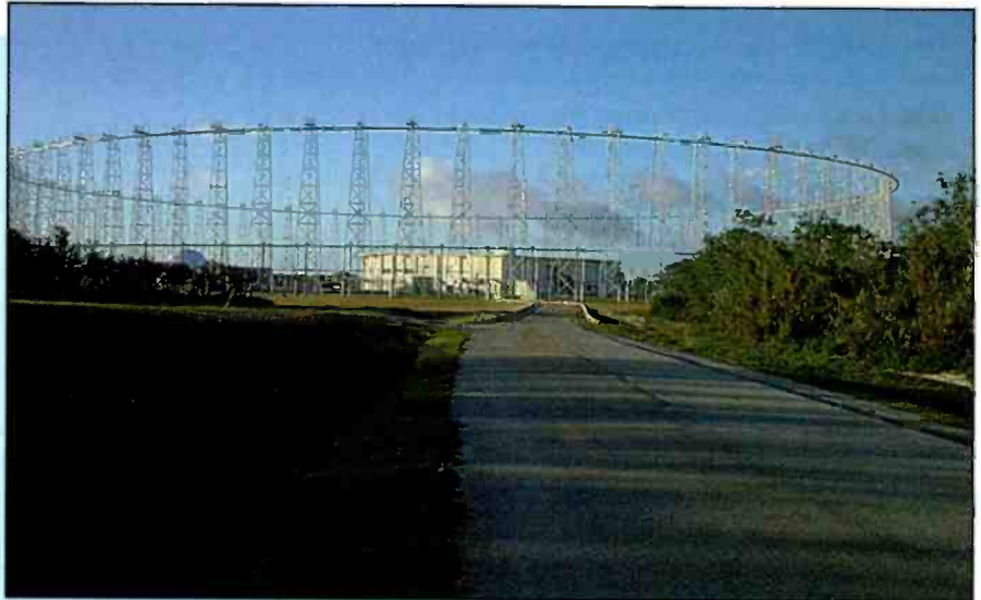
Before the advent of satellite-based navigation the U.S. Navy operated an extensive HF direction finding network. Pop'Comm reader, Fred Muller took this picture in May 2000. It shows the Wullenweber antenna located at the Naval Computer and Telecommunications Station on Guam. The station is now decommissioned and has been all but abandoned.
